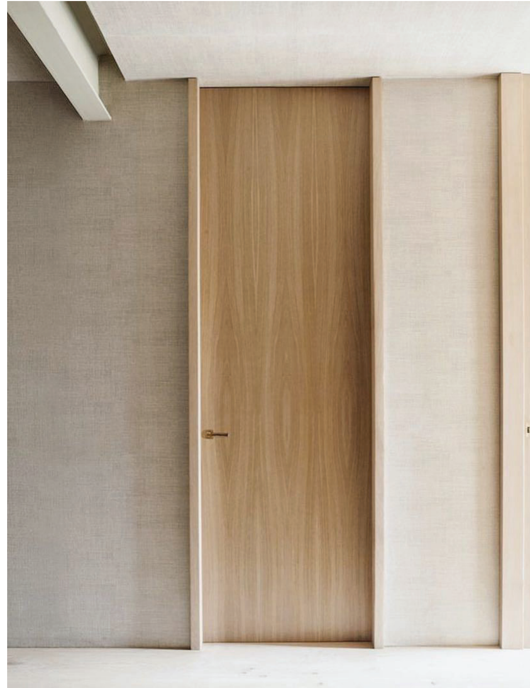
BLACK STAINED RIFT OAK SLAB WOOD DOORS WITH EXTENDED FLY-BY JAMBS FIXED PANEL ABOVE 8' HINGED DOORS TO EXTEND TO LID; FIXED PANEL TO MATCH FINISH OF DOOR PANEL BELOW
